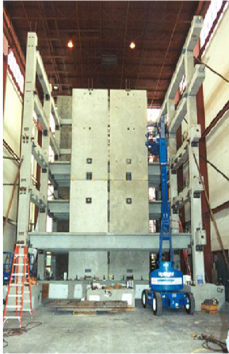
Figure 2.29 The jointed precast wall included in the PRESSS test building (Priestley et al. 1999)
